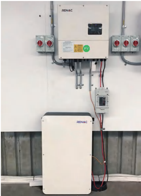
Residential Storage in Sydney Australia PV Self-consumption, 5kW hybrid inverter ESC5000-DS and 7.2kWh LPF battery
