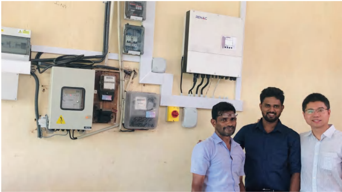
Residential Storage in Sri Lanka Solar+Storage, backup power, 20 units 5KW hybrid inverters ESC5000-DS
