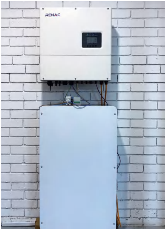
Residential Storage in Chelmsford UK 10 x 3.6kW/7.2kWh ESS for Firm frequency response, VPP, with hybrid inverter ESC3680-DS
