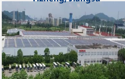
Roof PV Power Station in Honda Industrial Park
