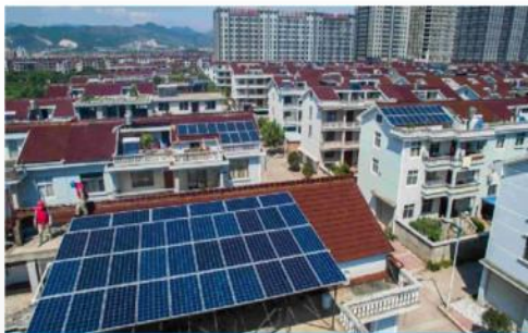
Residential PV Project in Dongyang, Zhejiang
