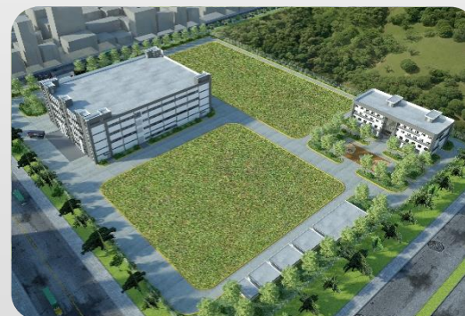
Manufacturing center Haiphong, Vietnam
