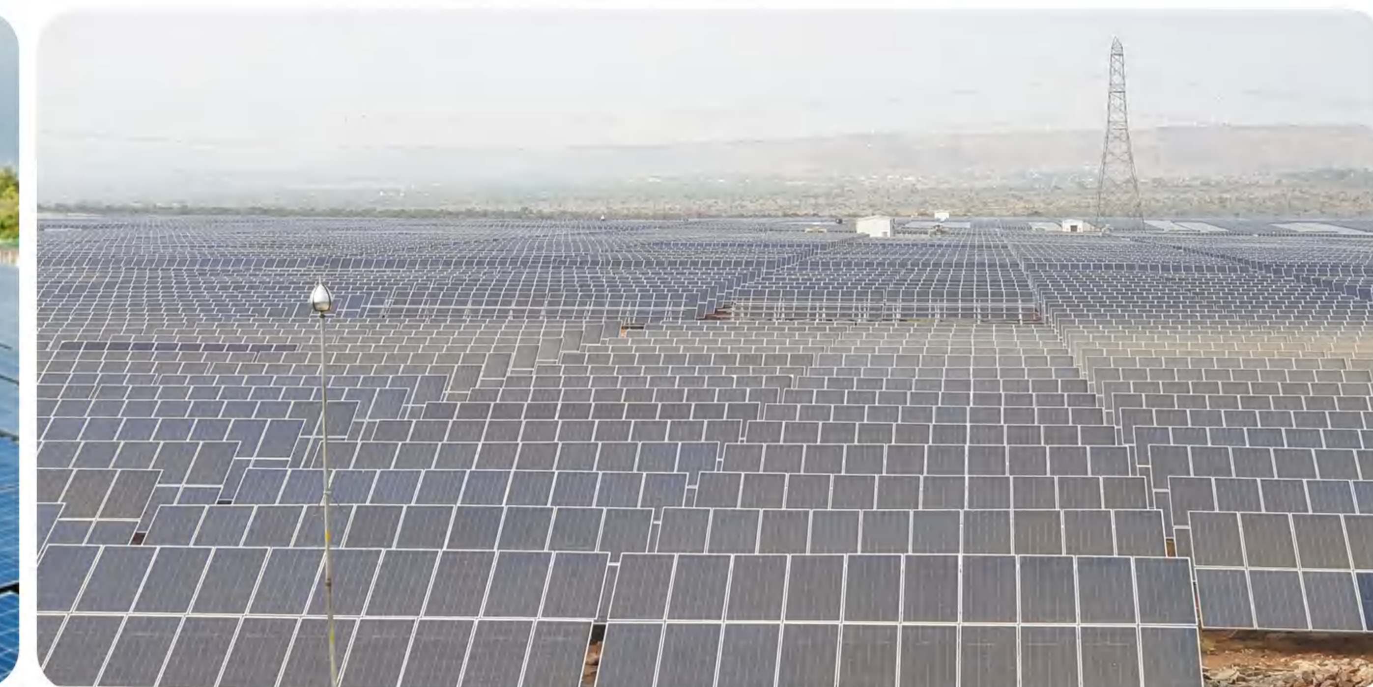
Installation of 2MW system in Hoceima, Morocco
