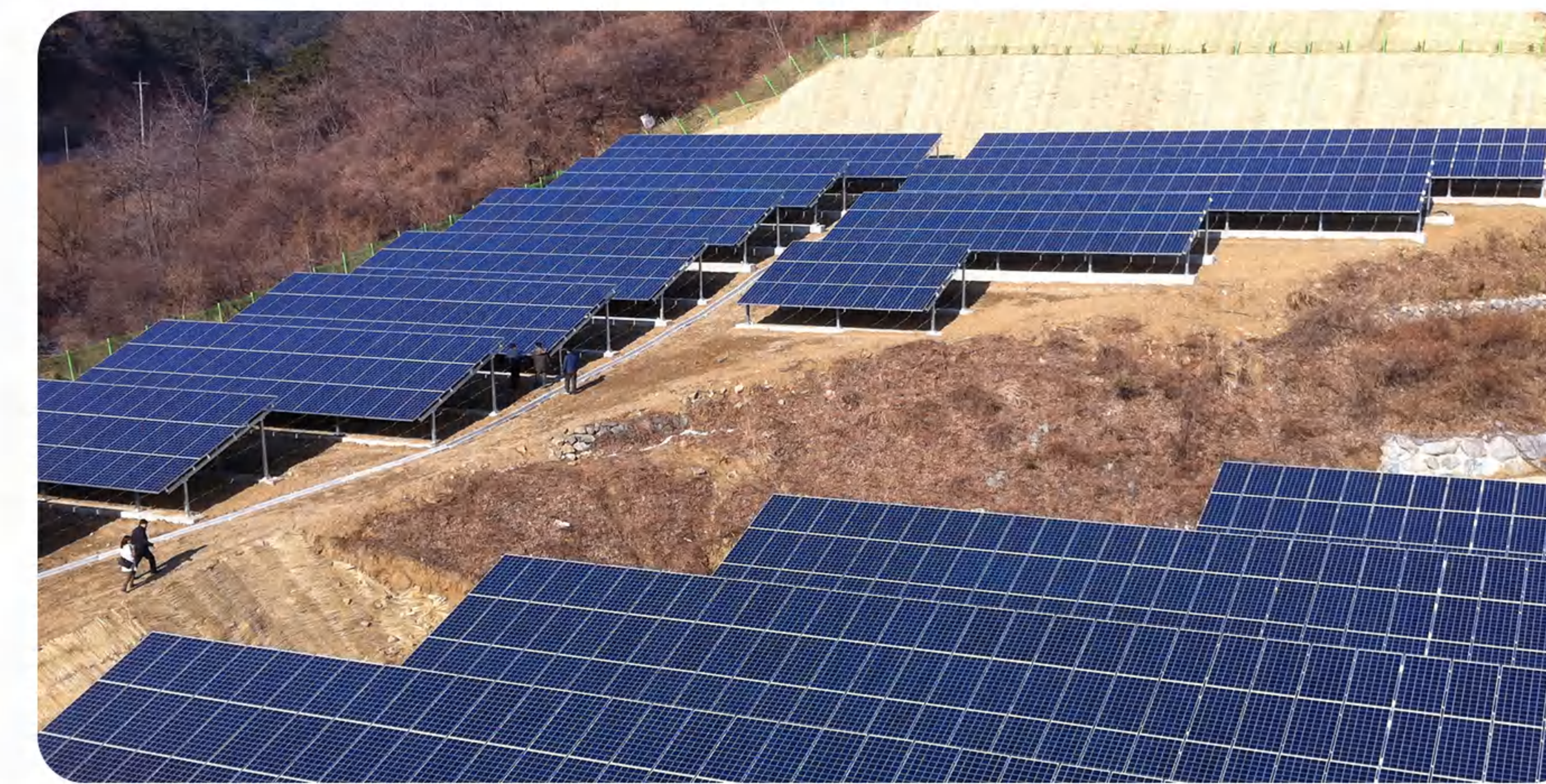
Installation of 2MW solar system in Amez Miz, Morocco
