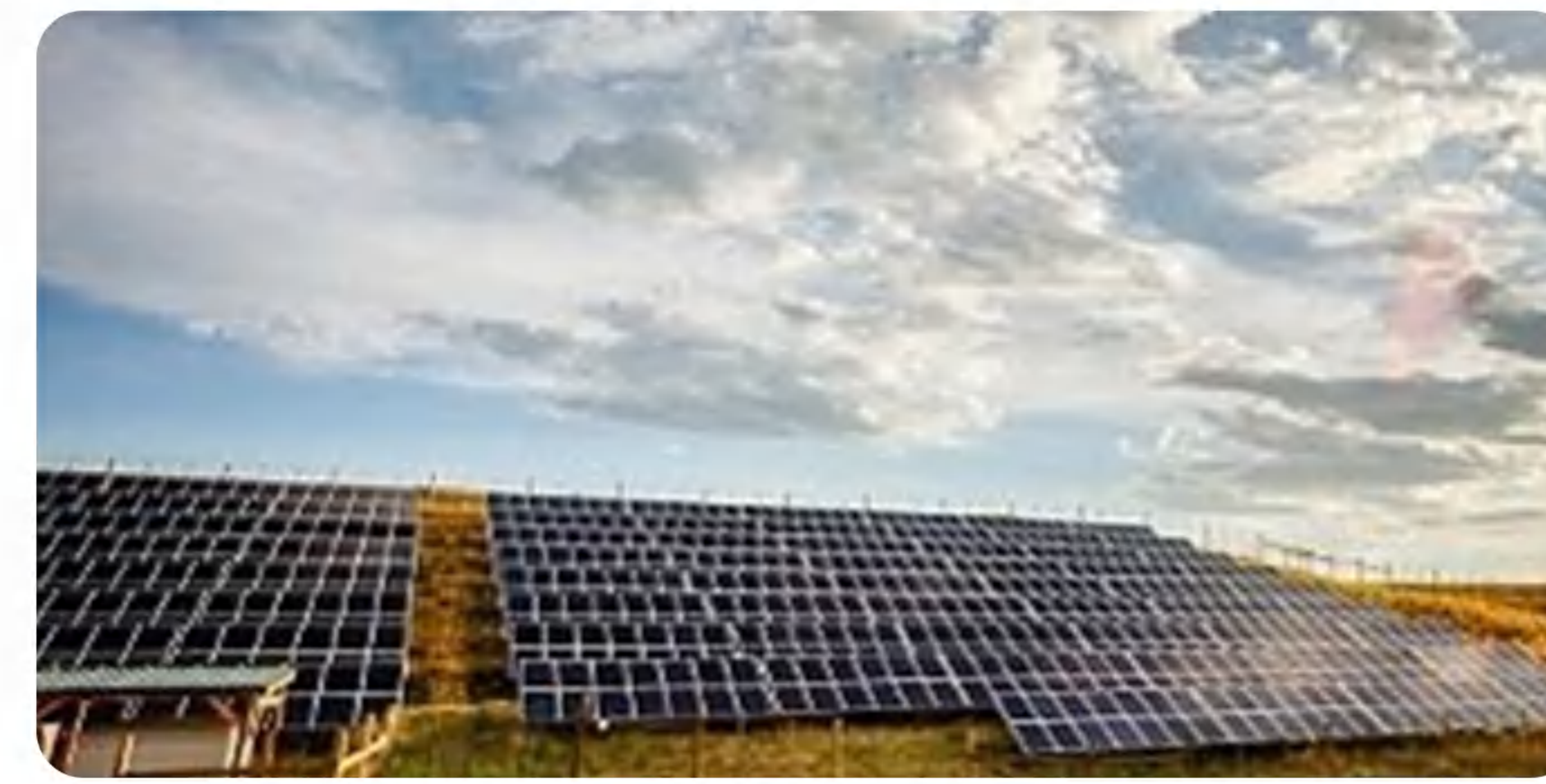
Vietnam Fu an Hua Hui 3MW ground photovoltaic project
