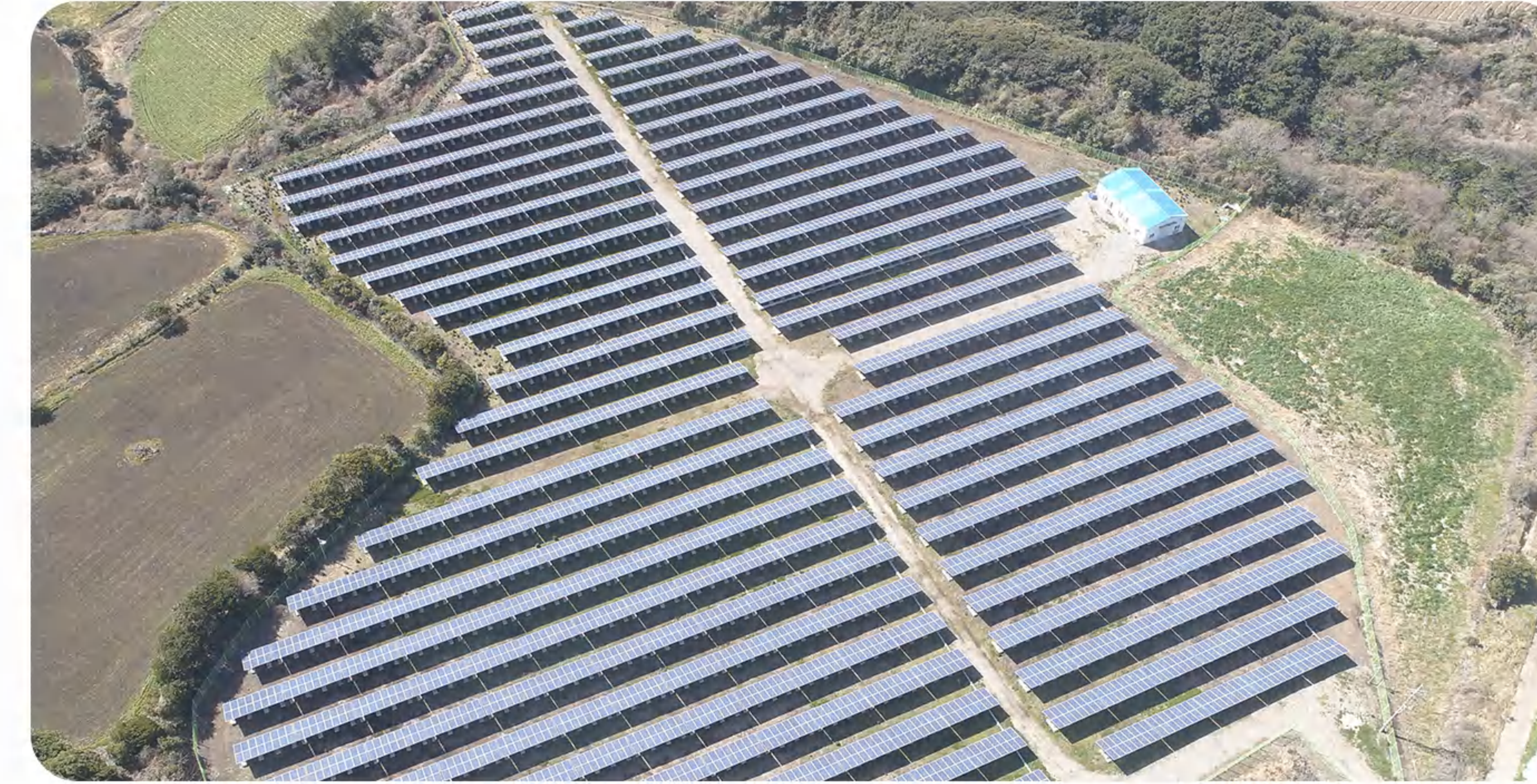
Installation of 2MW system
