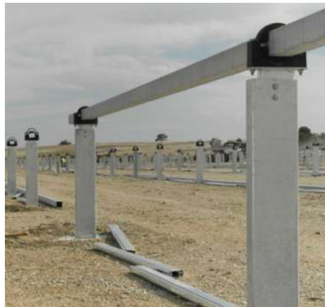
Image 34: Spherical bearings installed in Zuera 11 MW, Zaragoza
