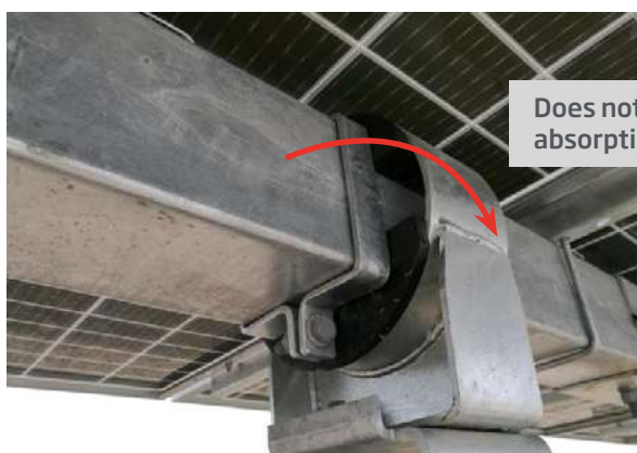
Image 16: Cylindrical bearing structure
